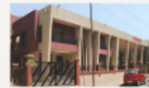
FIRE STATION - KOPERKHAIRNE
