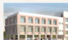
COMMUNITY CENTER - GHANSOLI
